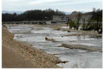
**Rheinfelden** - bypass with largest constructed reproduction habitats in Europe, pool type fish pass, vertical slot fish way.
