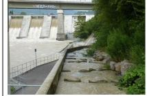
Wettingen at River Limmat, bypass channel with sections of vertical slot, pool type fish pass and habitats.
